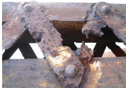
Fig 4 - Pitting corrosion occur on river bridge
