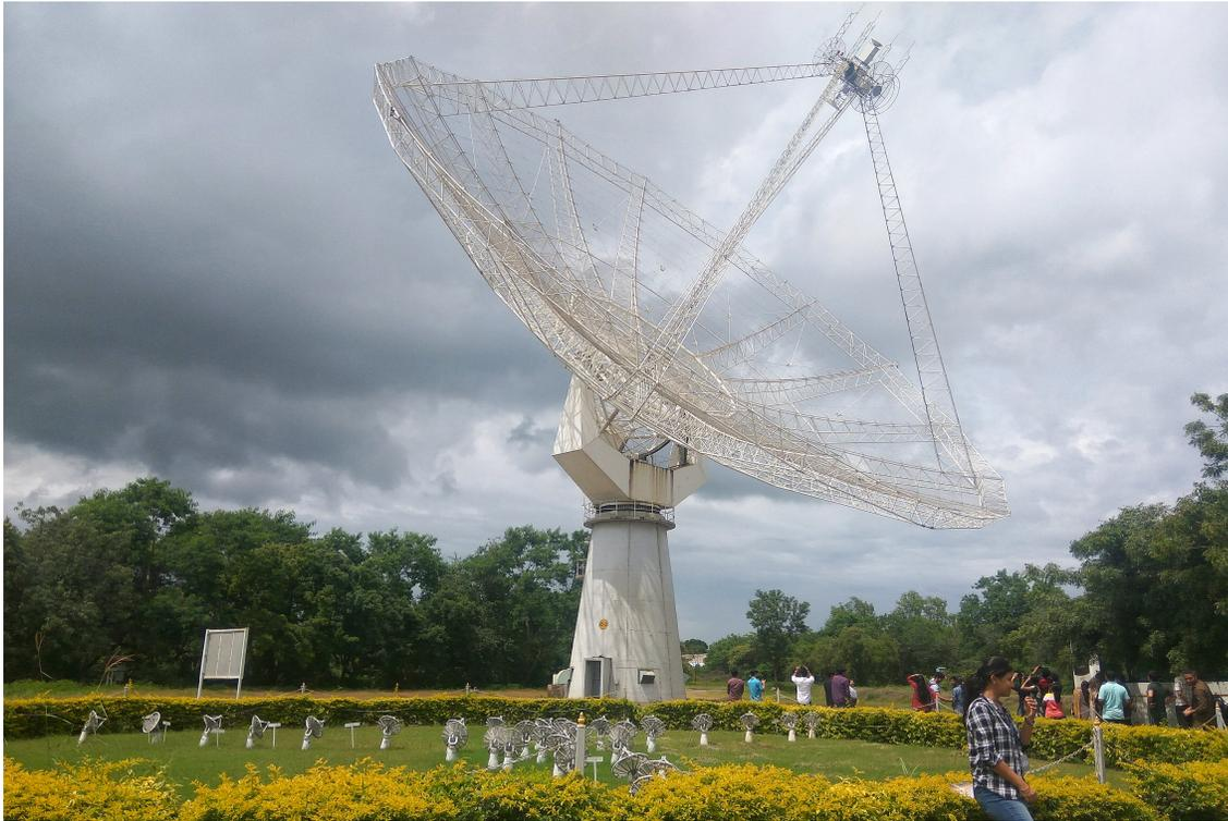
Figure 2.1: Antenna C3 of the uGMRT telescope, alongside a model of the array configuration. The antenna is 45 meters in diameter and is part of the central square. *Image Credit: Parul Janagal*
