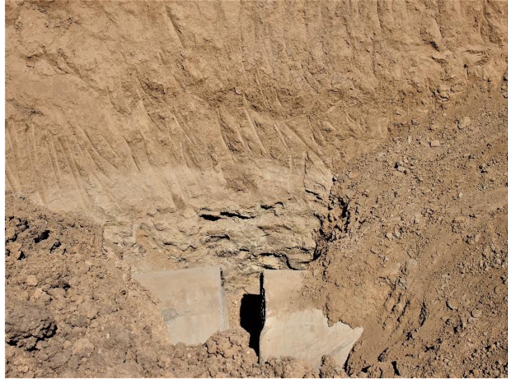
Photograph 18: Pipes laid had gaps in between
