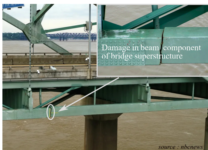
Figure 1.1: Damages on I-40 bridge superstructure
