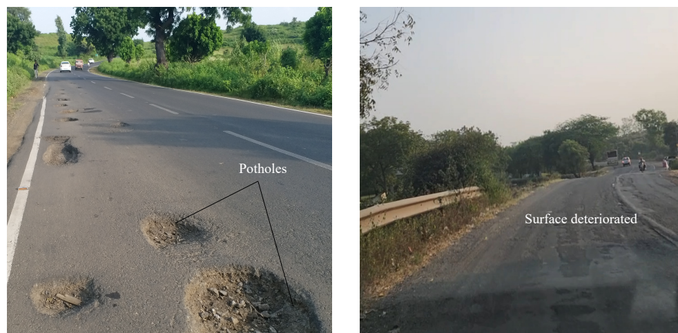
Figure 1.5: Different types of damages on road networks
