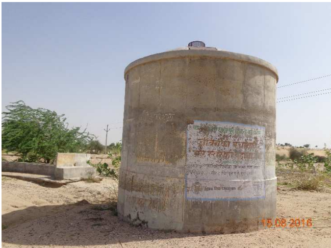
Here the picture shows a water box. Water from government is supplied to these tanks through pipeline during pre-monsoon period.
